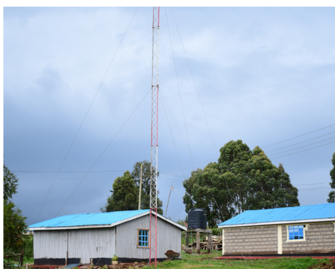
Figure 6: Ainabkoi FPO telecommunication mast
